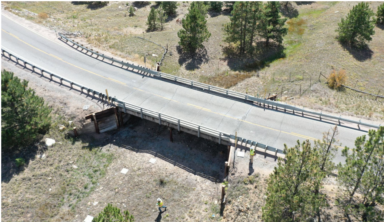
Picture 1 – Bridge J-14-C General Location
