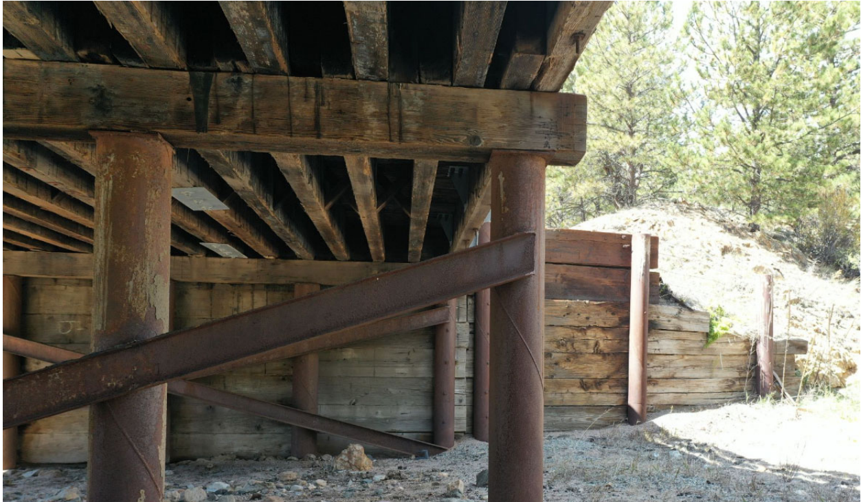
Picture 2 – Girders, Pier, Wingwall
